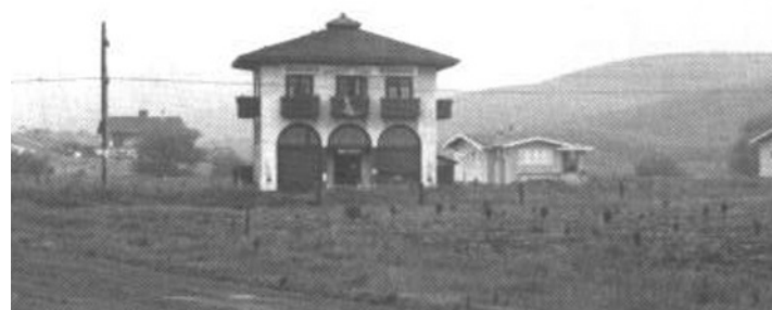
Photo courtesy of Canyon Construction
