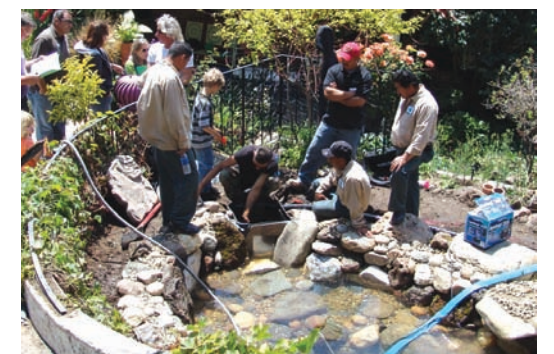
Installing the 4000 gallon per-hour pump
