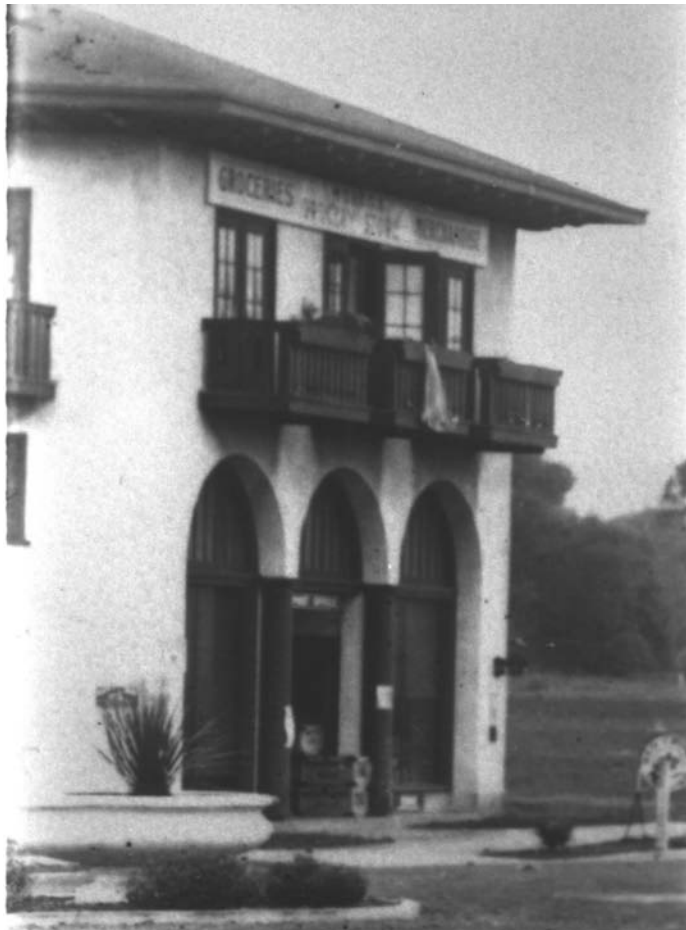
Historical picture of the Moraga Barn
