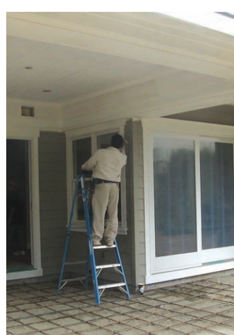
Energy-efficient windows being installed Photo provided by Kattenburg Architects
