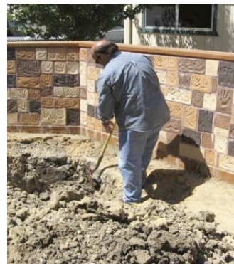
Excavating the wall
