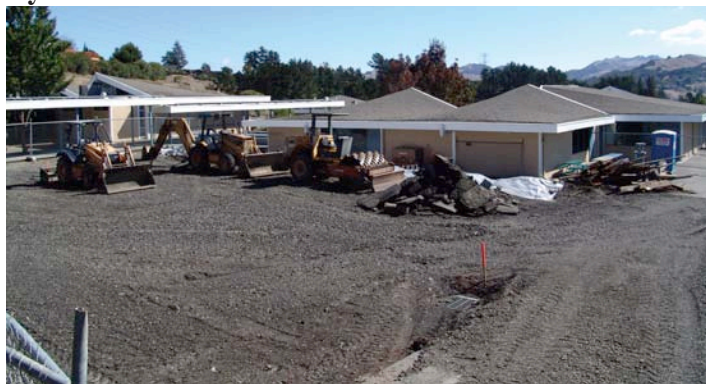
Los Perales, under construction
