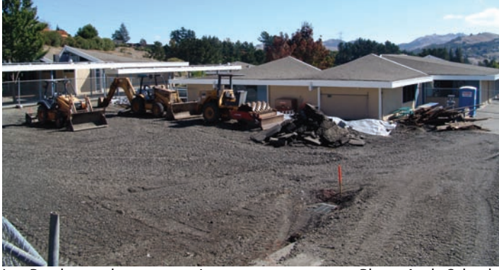
Los Perales, under construction
