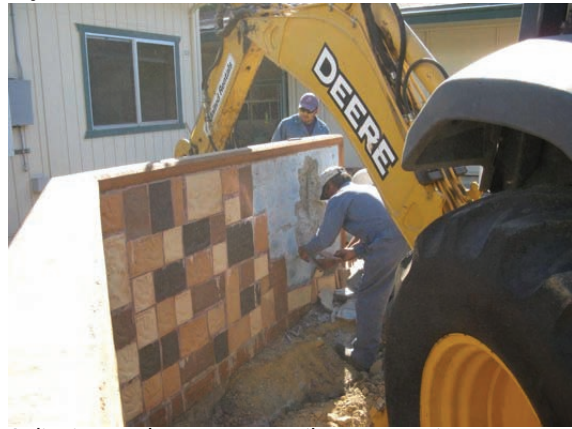
A district employee removes tiles one at a time
