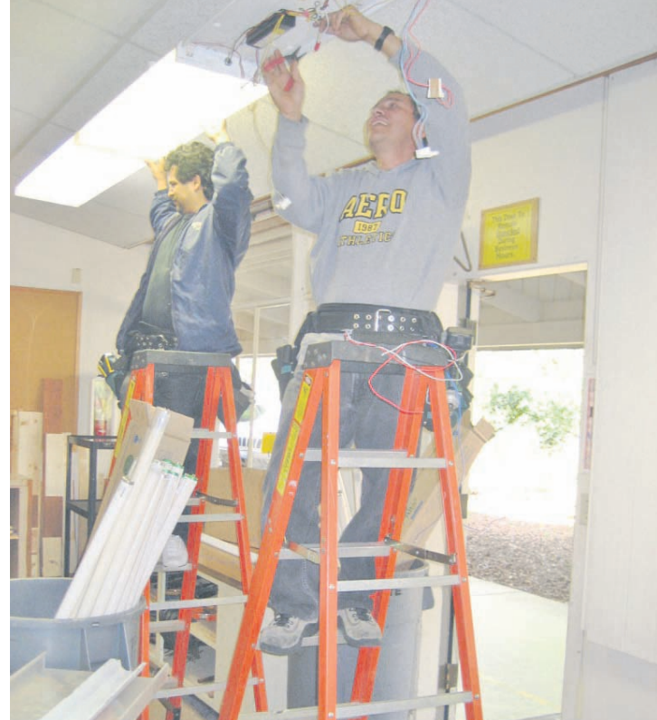
Workers installing more energy efficient lights Photo courtesy of Jennifer Russell
