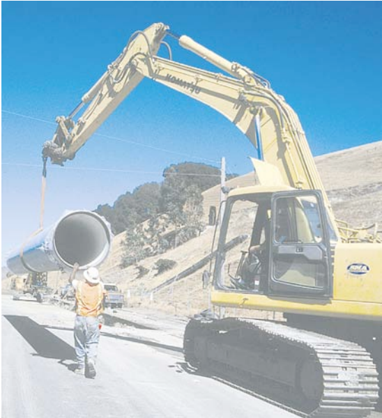
Big equipment for big pipes is coming in town Photo provided
