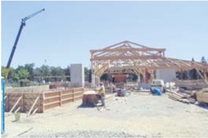
Construction site on Mt. Diablo Blvd.
