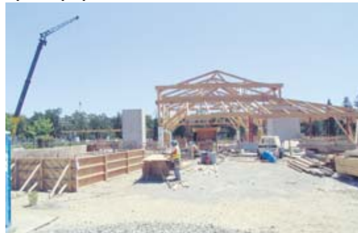
Construction site on Mt. Diablo Blvd. Photo Andy Scheck
