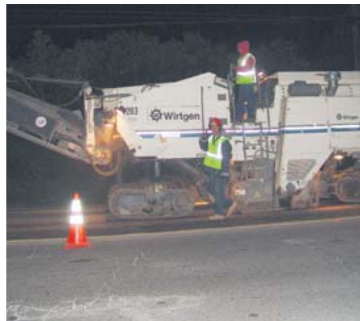
Night work on Moraga Way
