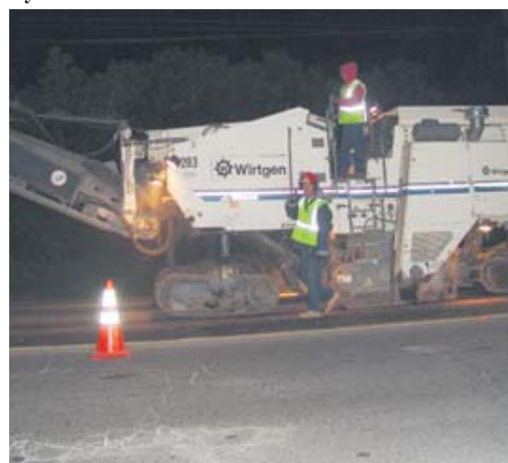
Night work on Moraga Way
