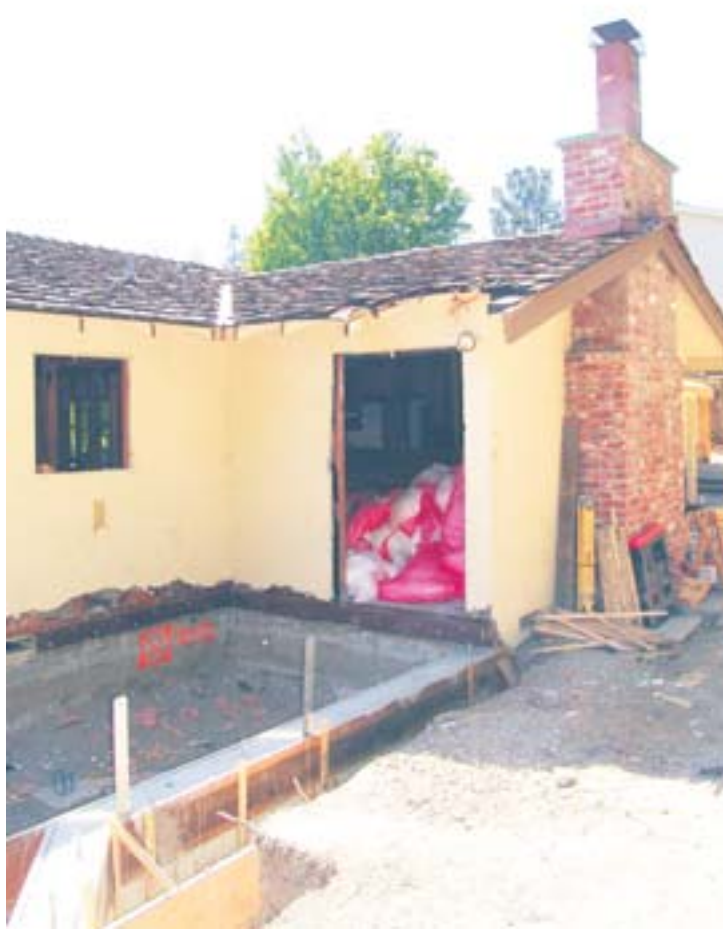
Ryerson residence under construction
