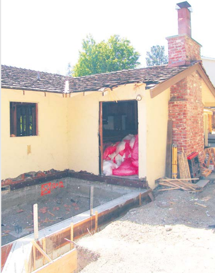
Ryerson residence under construction
