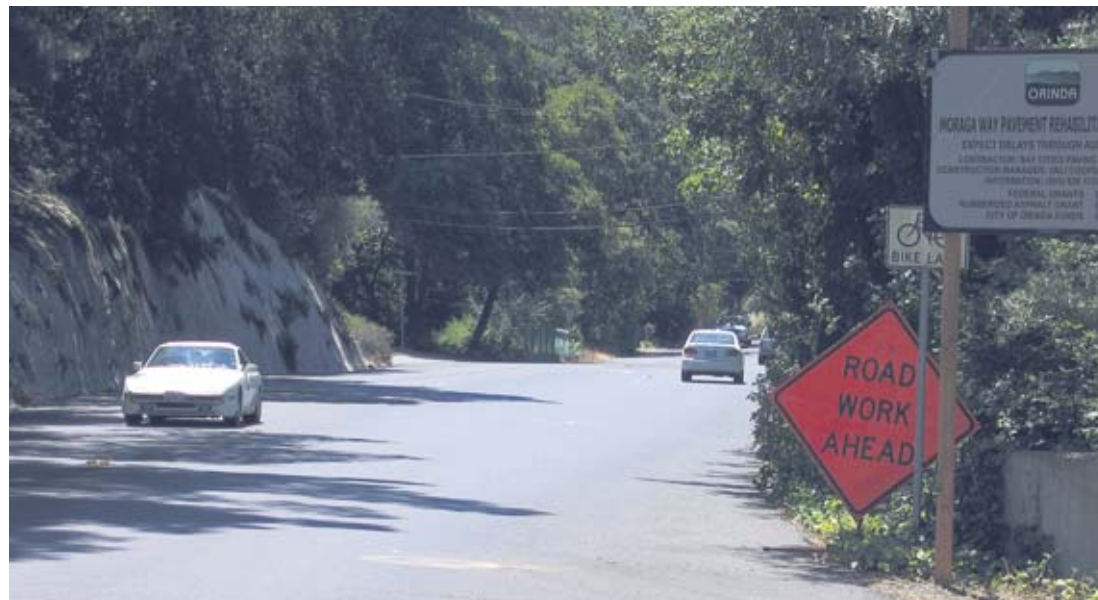
View of the new and improved Moraga Way
