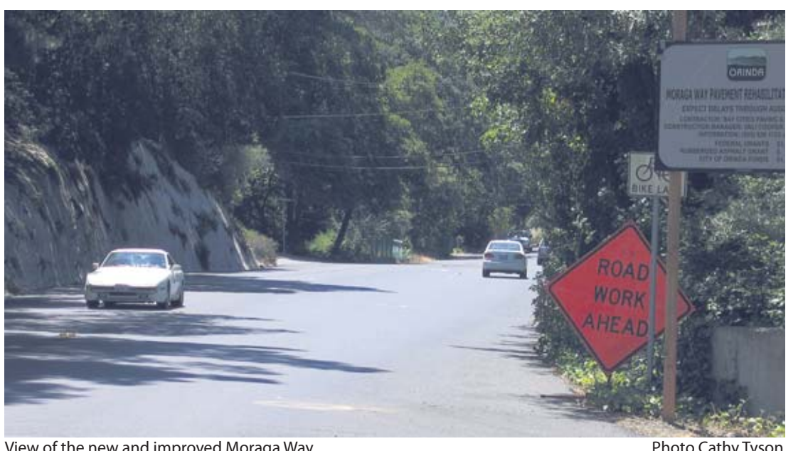
View of the new and improved Moraga Way Photo Cathy Tyson
