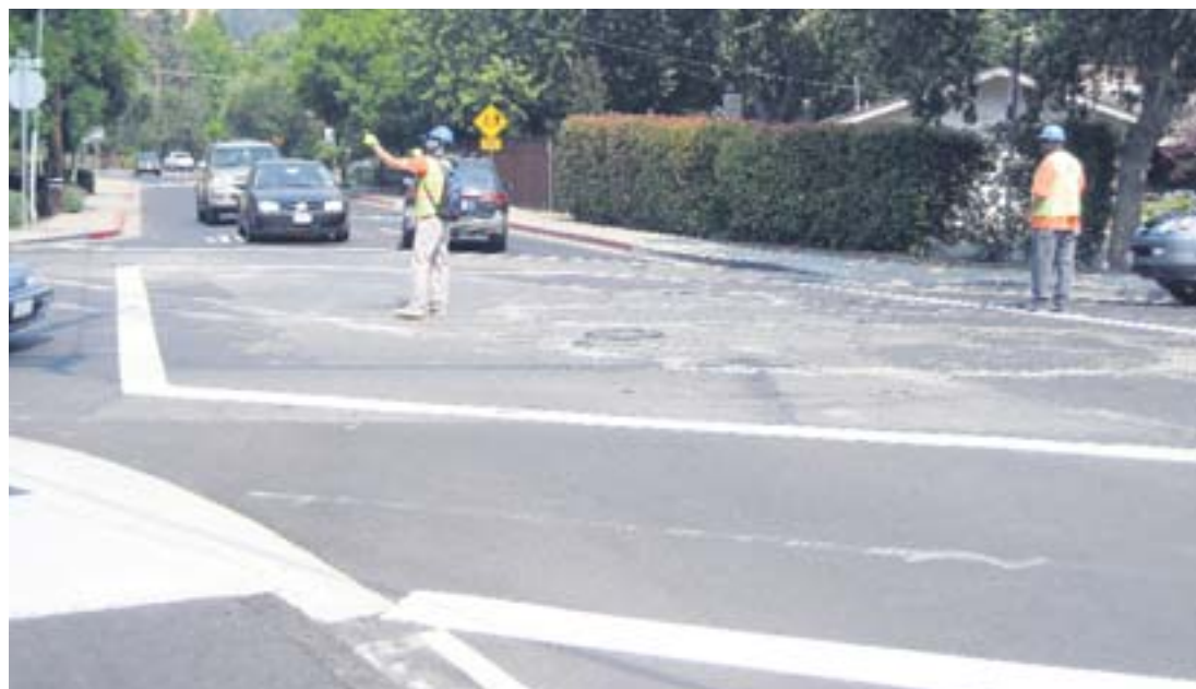
Mountain Cascade flagmen directing traffic in 104 degree heat
