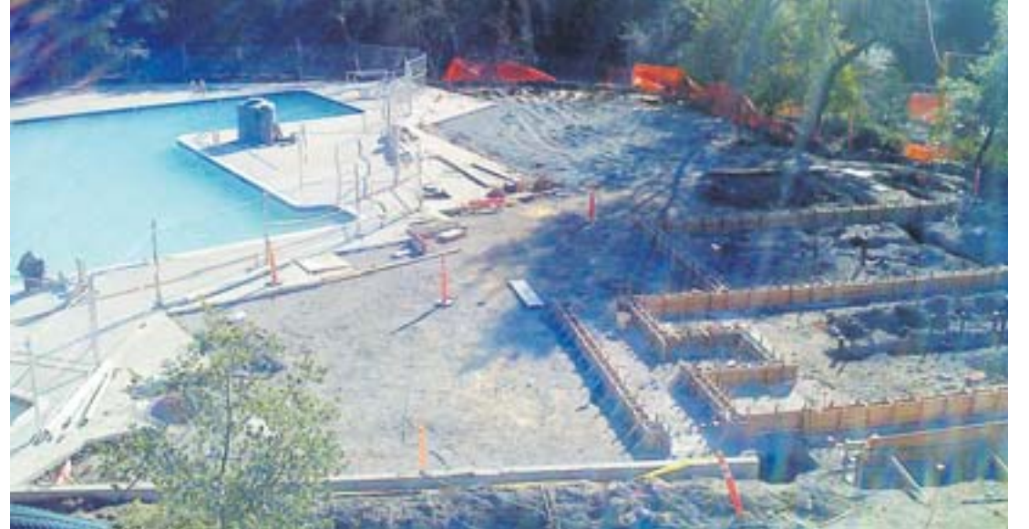
View of the “Rancho” main clubhouse, still under construction
