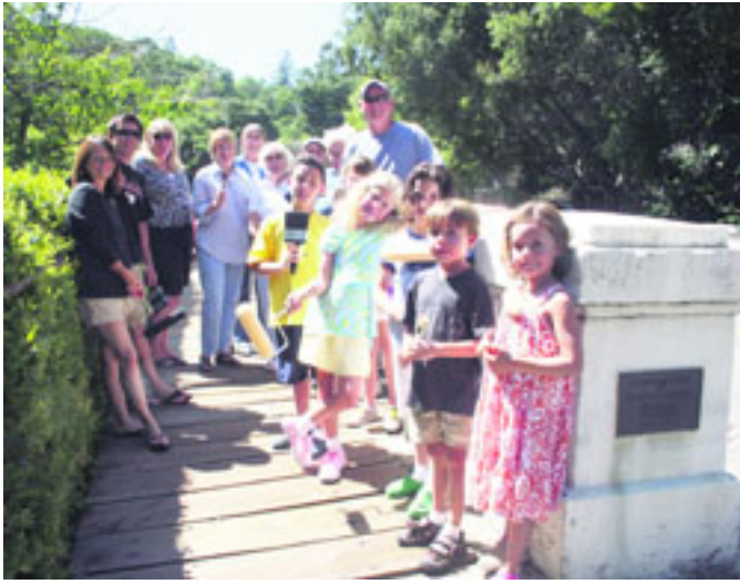
Members of the Orinda Historical Society and friends preparing for the bridge restoration on Saturday, August 1st. Photo A. Firth
