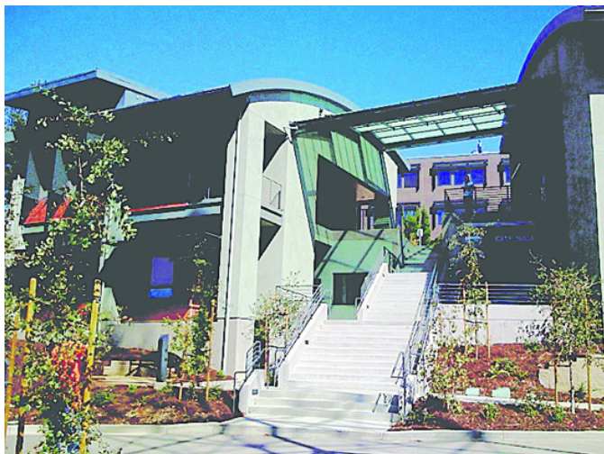
Orinda City Hall exterior, west side. Photo Tod Fierner
