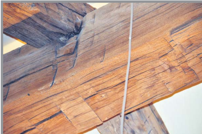
100-year old reclaimed wood ceiling beams in Sawczuk's kitchen
