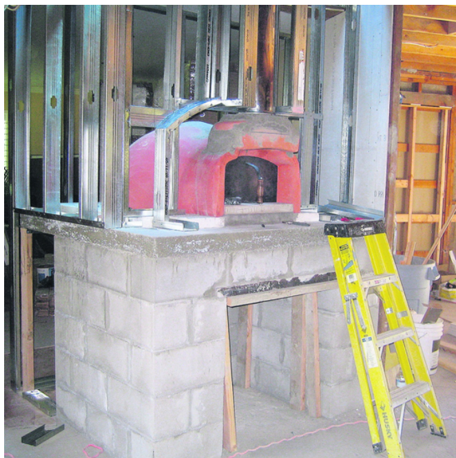
Building the pizza oven Photos Pat Geoghegan
