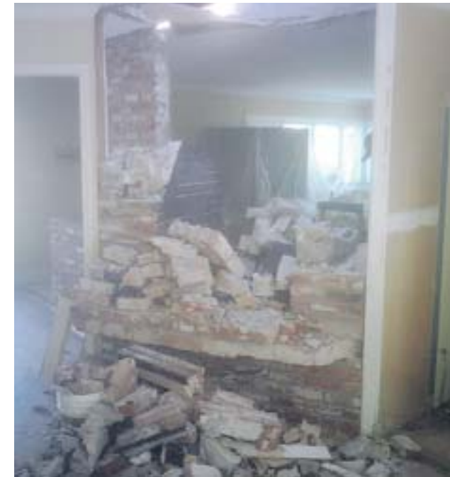
The Keough's old fireplace was demolished
