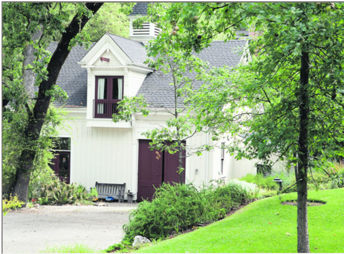
The former guest cottage was remodeled, keeping a part of the original cottage and building an addition.
