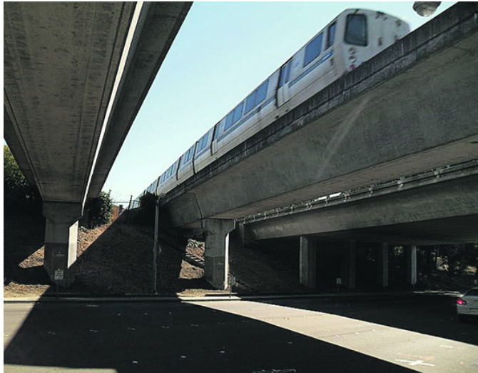
Bart bridge over Oakhill Road Photo Cathy Tyson
