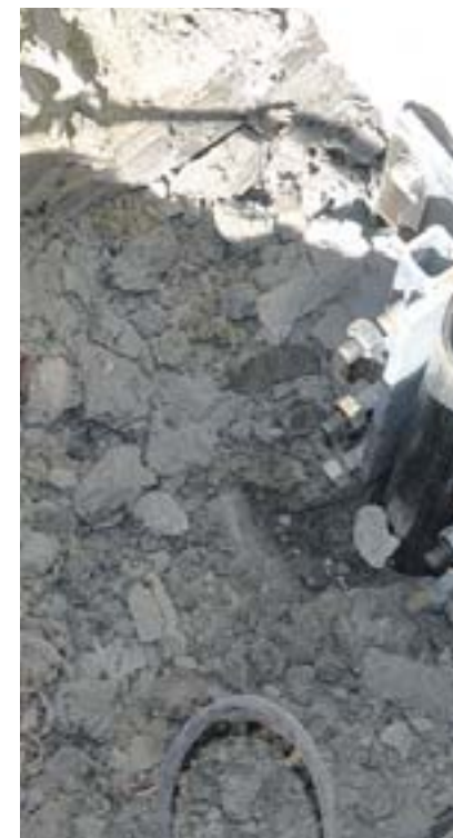
Installed pier pipe
