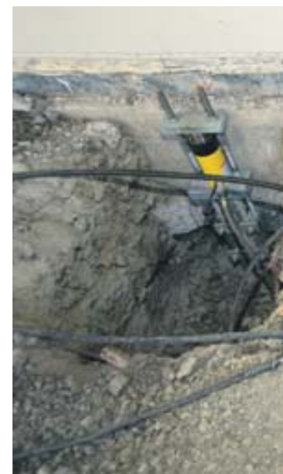
Lift set up
