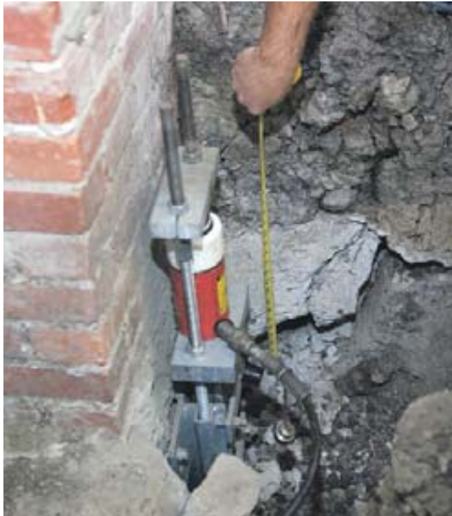
Measuring the progress
