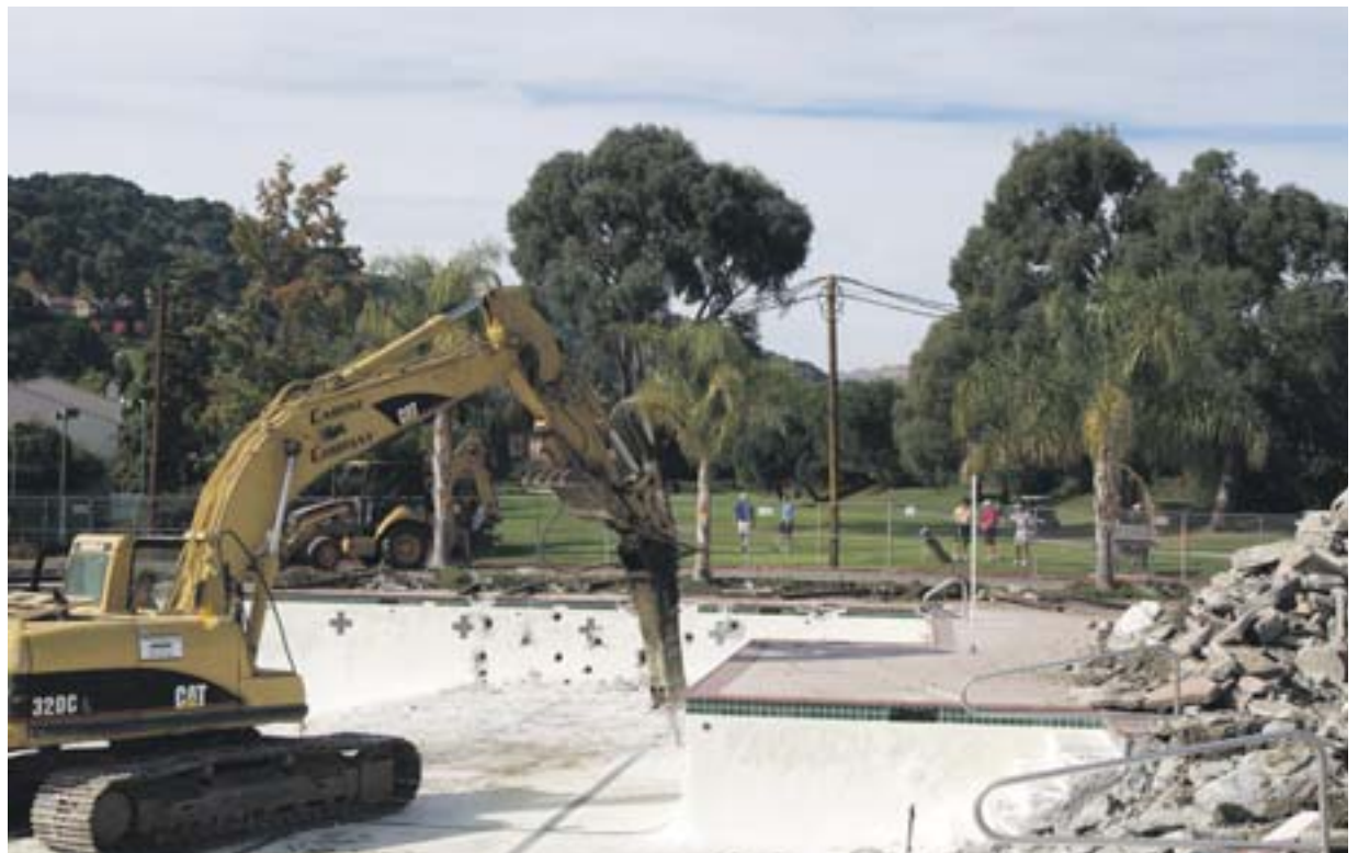
Old concrete will be recycled and reused at the site
