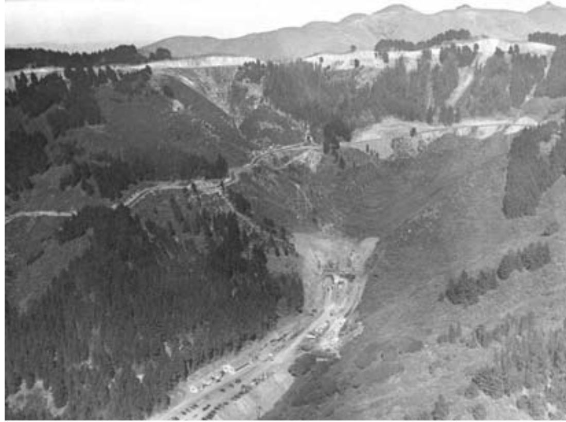
Construction of bores 1 and 2.
