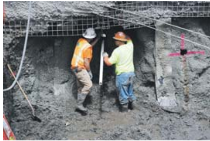
Workers in the mud
