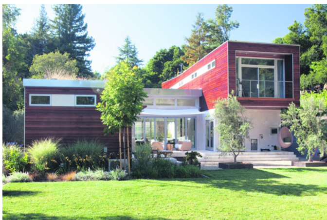
View from the backyard of Remick's sustainable home. Photo Mariko Reed
