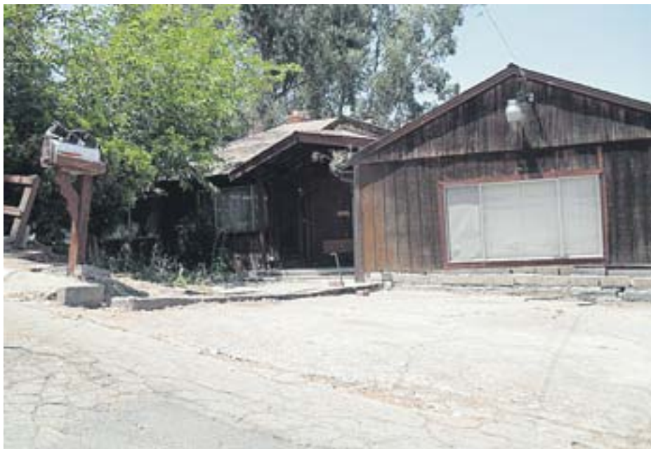
Exterior of Ruth Court home in Lafayette before remodel.
