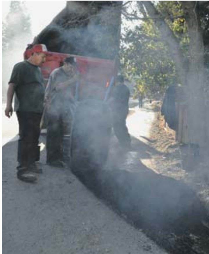
Hot steaming asphalt comes off the Lucas truck Photo Andy Schreck
