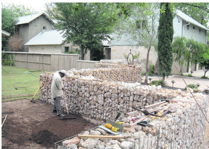
Building a gabion wall Photo provided
