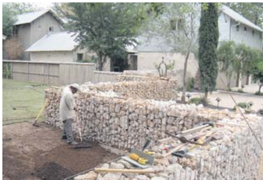
Building a gabion wall
