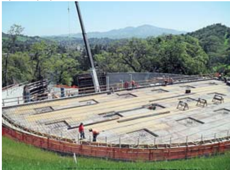
Crews working on the partially completed Highland Reservoir last week.
