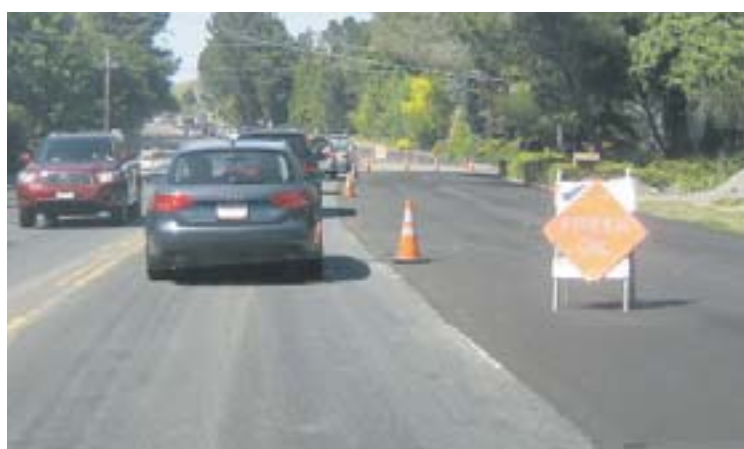
Long lines of cars as the road is repaved
