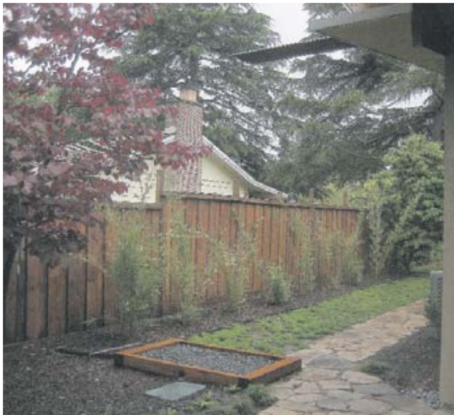
Downspouts direct water to sand basin
