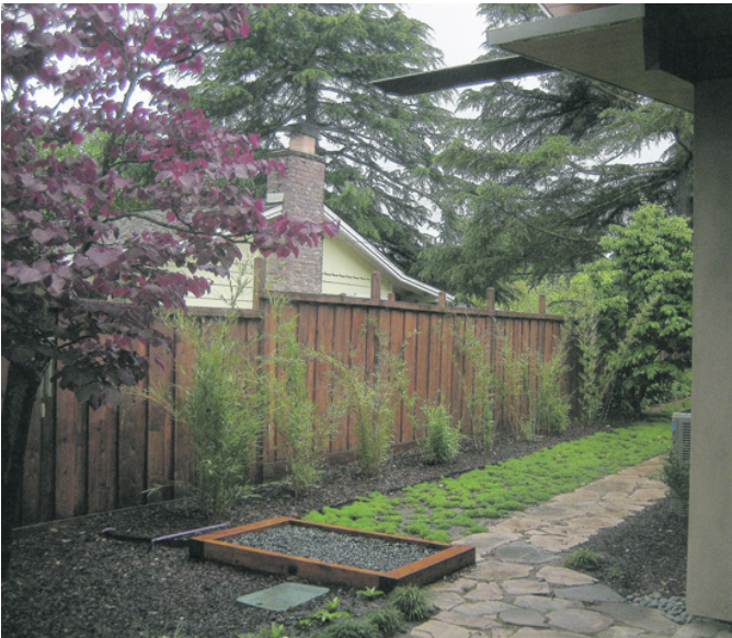
Downspouts direct water to sand basin Photos Sophie Braccini
