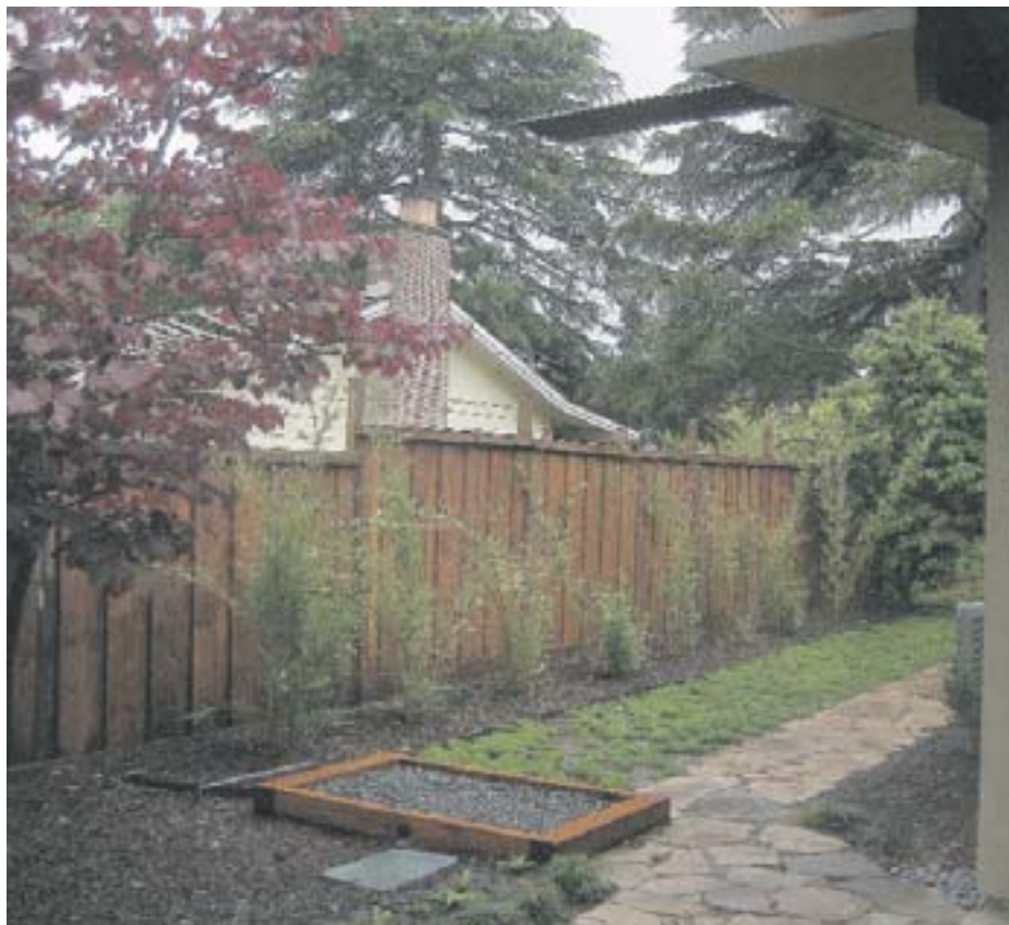
Downspouts direct water to sand basin
