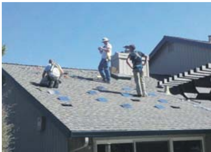
Measuring the roof
