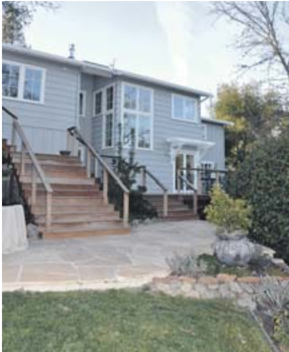
Wrap-around windows (center) provide bright natural lighting for the interior staircase off the family room.
