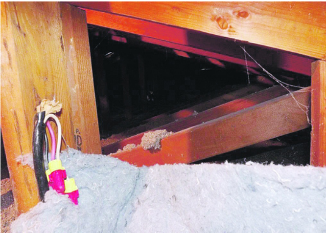
Check on electrical wires
