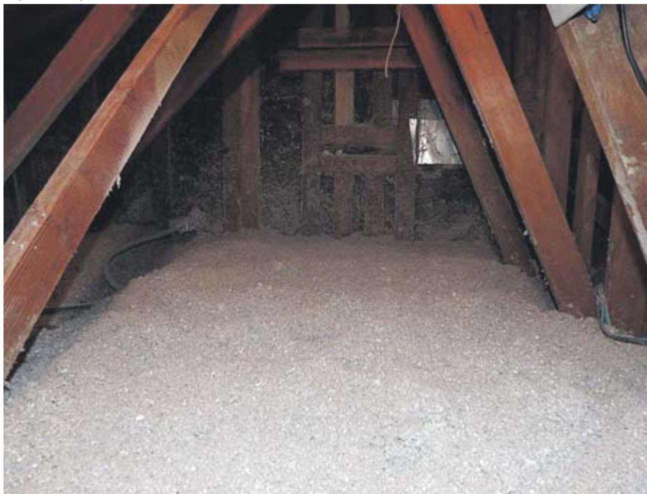
Replaced new insulation
