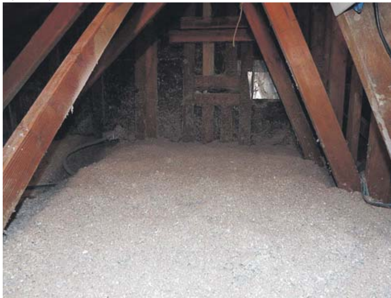
Replaced new insulation
