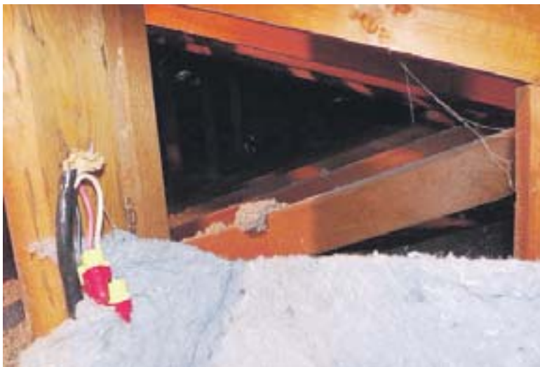
Check on electrical wires
