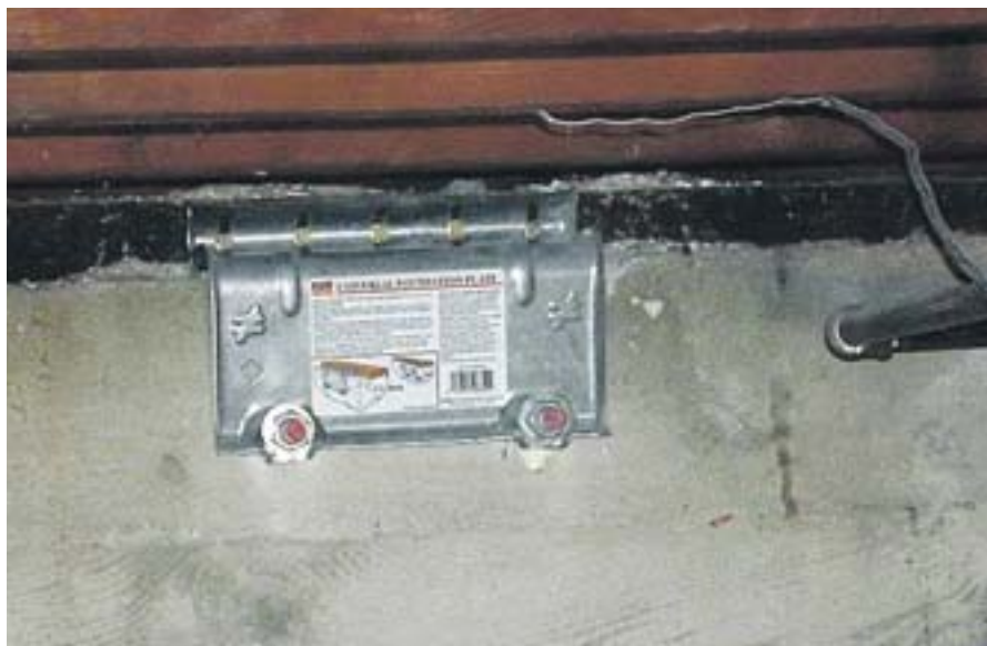
Foundation plate brace, connects concrete foundation to mud sill
