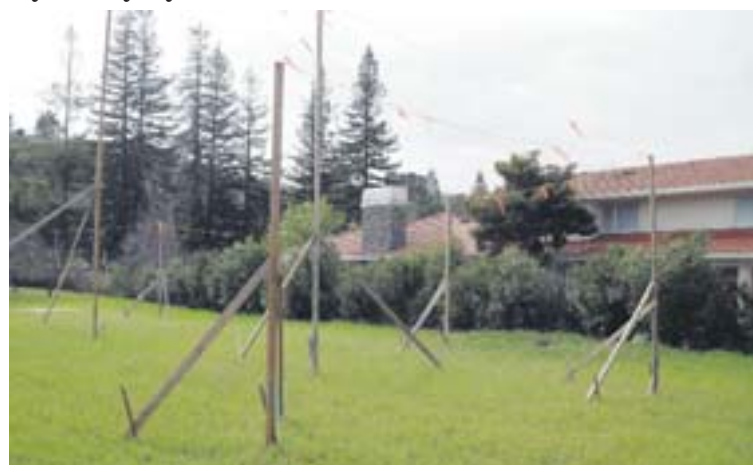
Story poles of proposed home on Las Huertas Road. Photo C. Tyson
